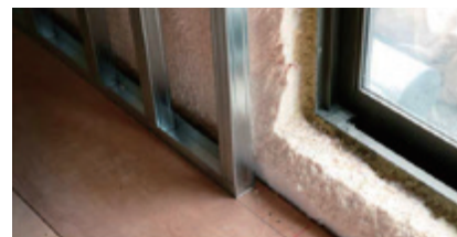
Urethane foam insulating material with roughly twice the thickness of the original insulation
